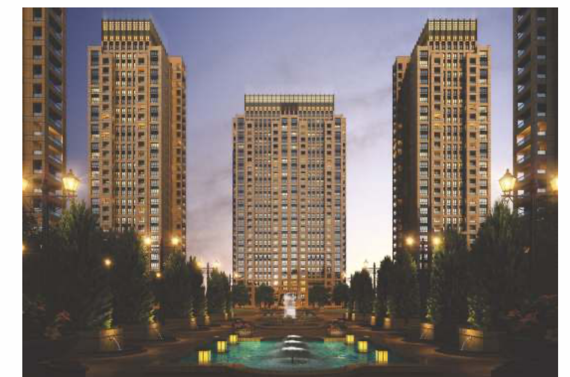
NOBLE AYRA, NEW DELHI ONGOING
